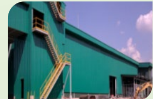
Solid Treatment Plant
